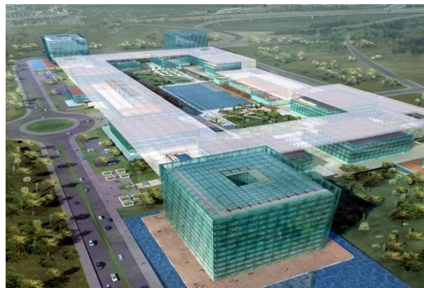
Large Office Complex
