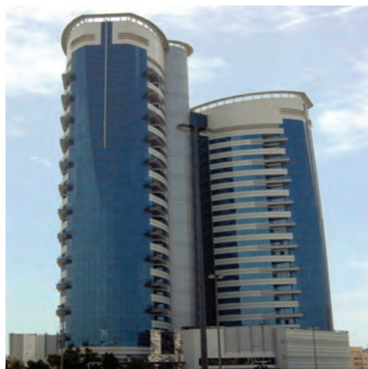
MANKHOOL TOWER, DUBAI
