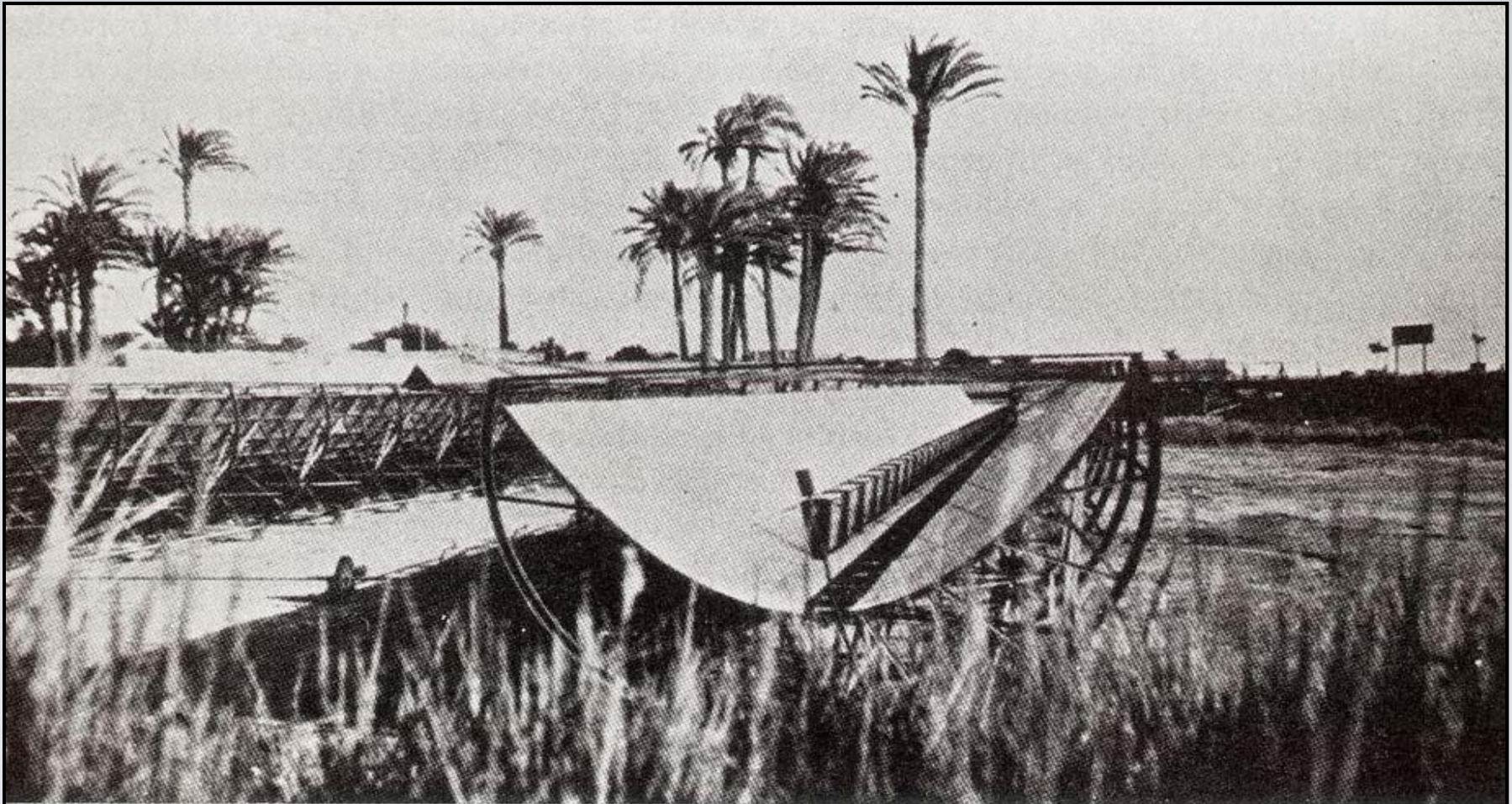
Fig. 1.9 Detail from the north of the long parabolic-cylinder mirror collectors used in the human-Boys system. Note the hoops on which the mirror was tilted to follow the sun.
